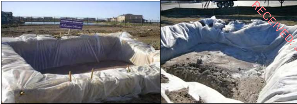
Plate 4-3 Concrete washout area
