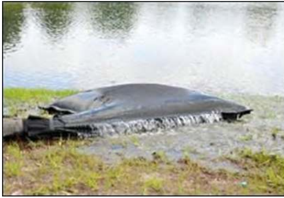
Plate 4-5 Silt bag with water being pumped through
