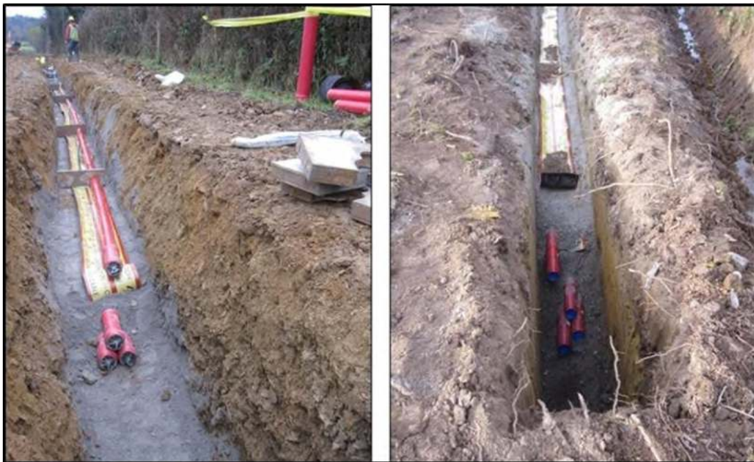
Plate 4-7 Standard Cable Trench View
