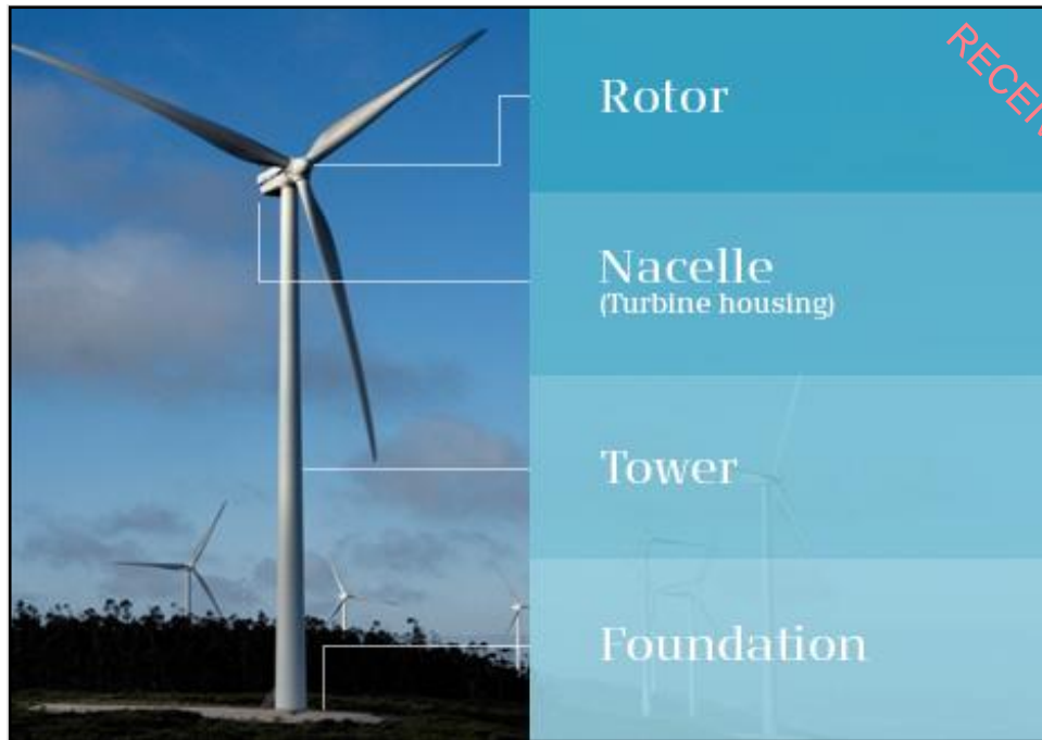
Plate 4-1 Wind turbine components
