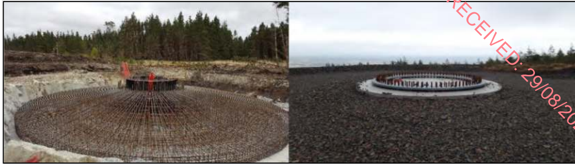
Plate 4-2 Turbine 'Anchor Cage' and finished turbine base
