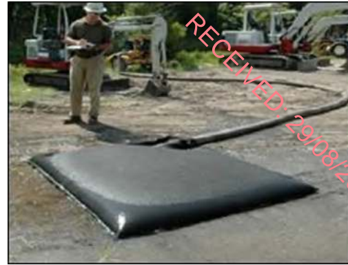
Plate 4-6 Silt bag under inspection
